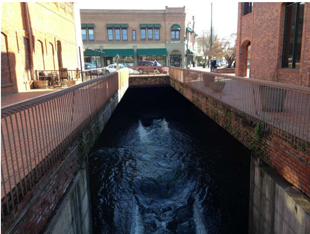
Figure 2.11-2. Daylighted Portion of Mill Creek (RM 7.2), Intersection of 1st and Main St.
