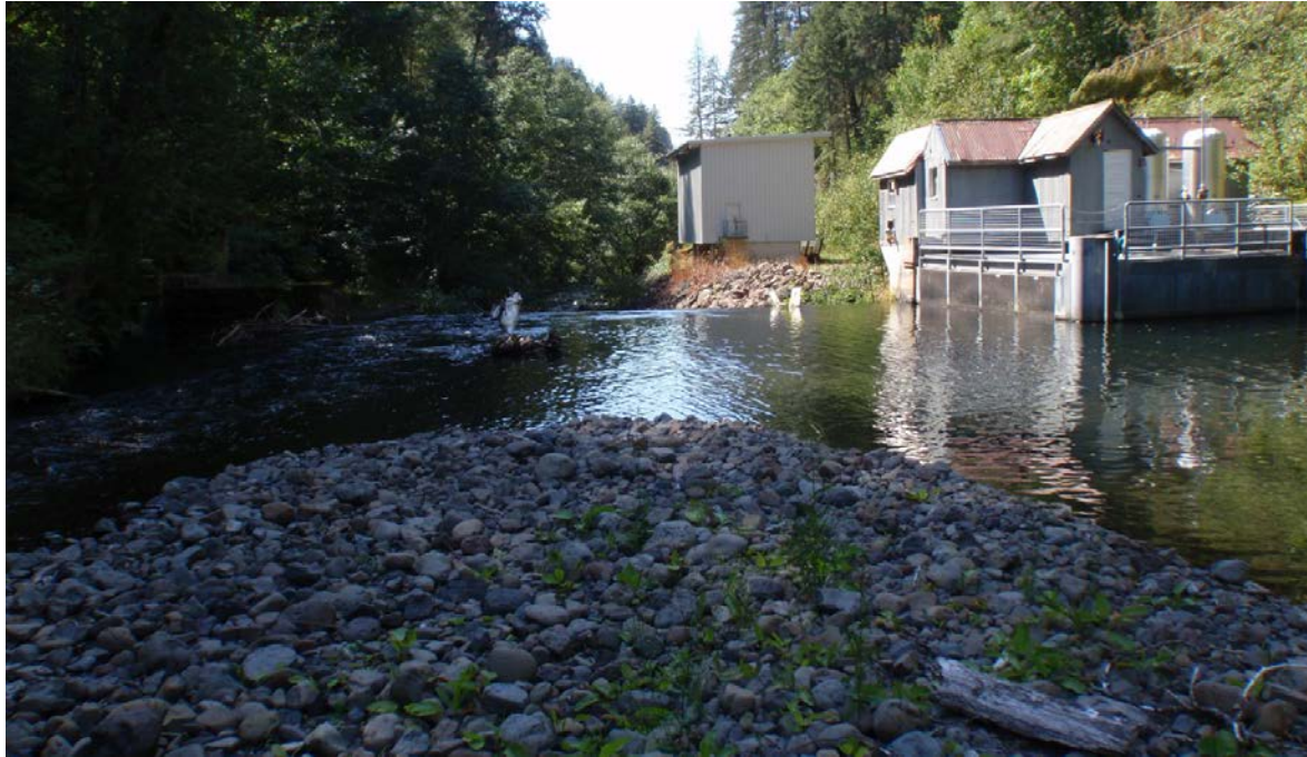
Figure 2.8-30. Habitat Conditions in the Upper Watershed by the Pump House
