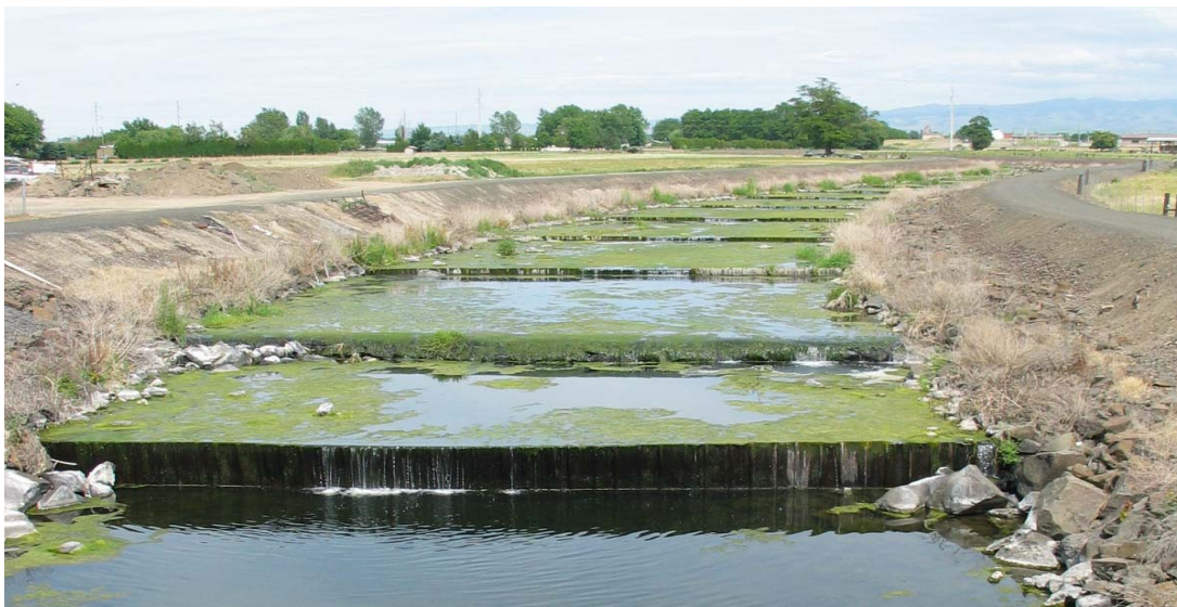
Figure 2.8-25. Flood Control Sills in Segment 2
