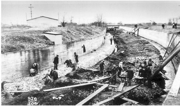
Mill Creek Channel Construction (Photo Source: USACE)
