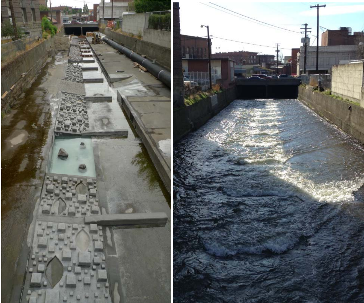
Figure 2.8-26. Corrective Baffles Upstream of the Underground Portion of Mill Creek Channel, at Construction (9/2014) and at Winter Flows (2/2016)
