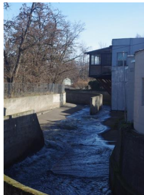
Building overhanging the Mill Creek Channel
