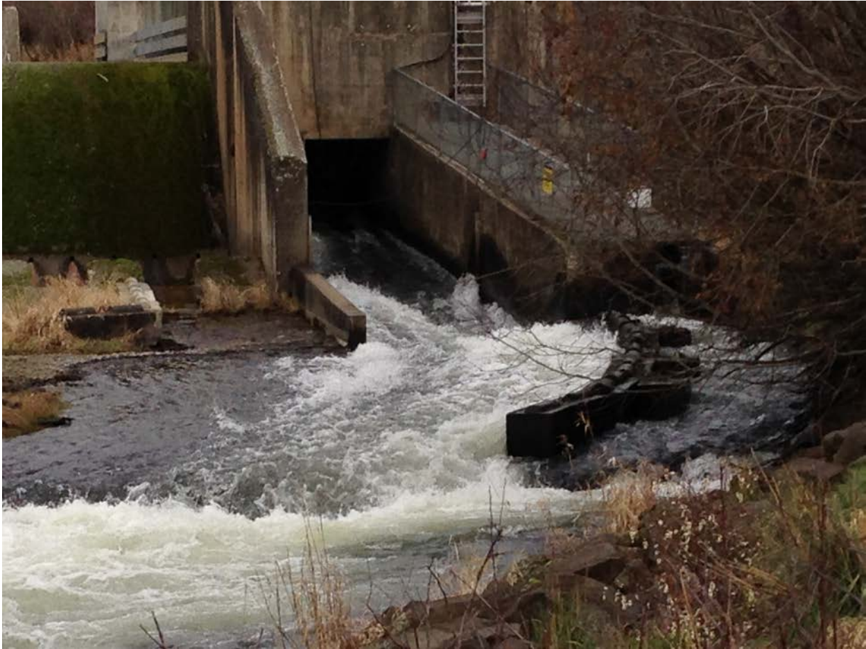
Figure 2.8-32. Bennington Diversion Dam low-flow outlet on left, fish ladder mouth on right.
