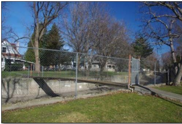
Pedestrian Bridge – Alder St. to Whitman Campus
