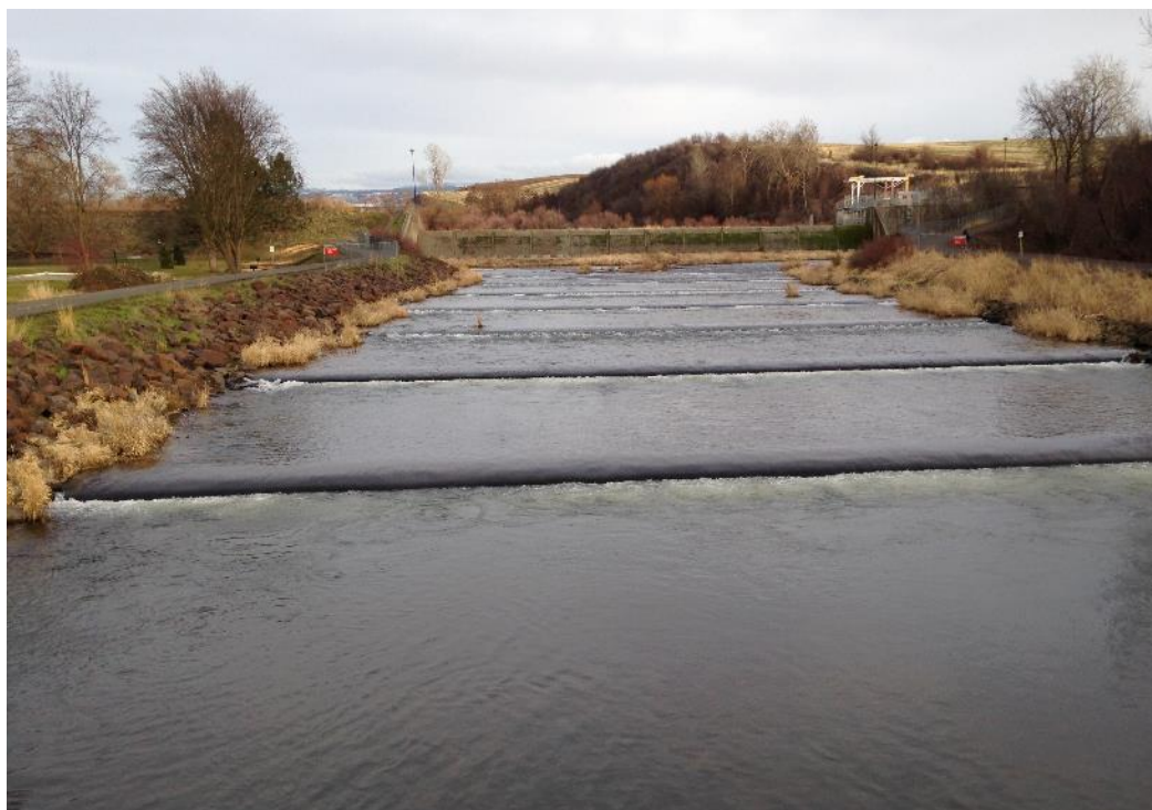
Figure 2.11-6. Mill Creek just below Bennington Diversion Dam (RM 11.4), Facing Upstream (Trail on Left)
