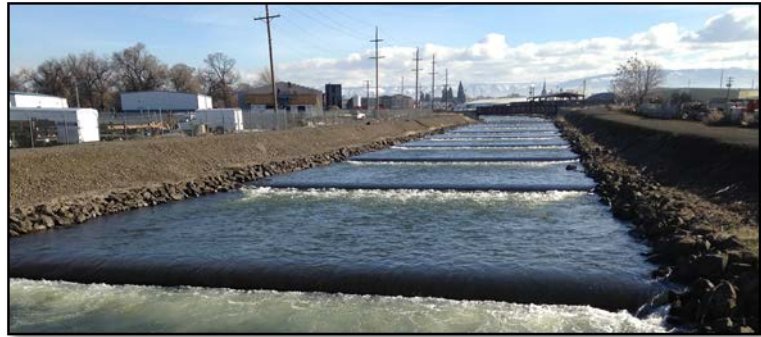
Mill Creek Segment 2 from 13th Street Looking Upstream at Railroad Bridge
