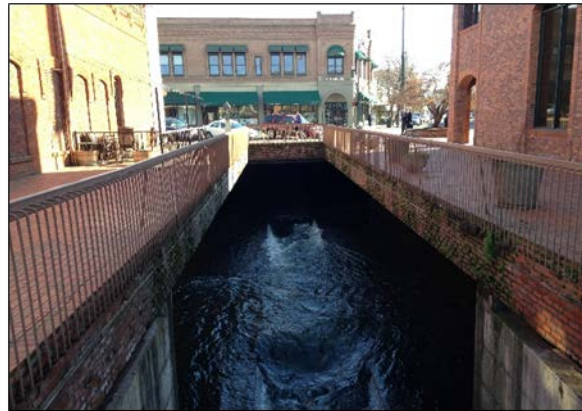
Exposed portion of underground channel off Main St.
