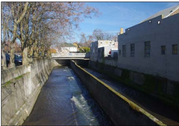
Channel looking upstream towards Palouse St.
